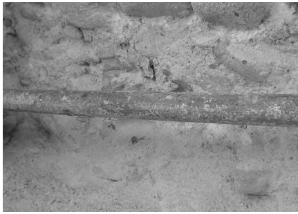
Fig. 12 Photograph of a reinforcing bar with little corrosion (level A)
