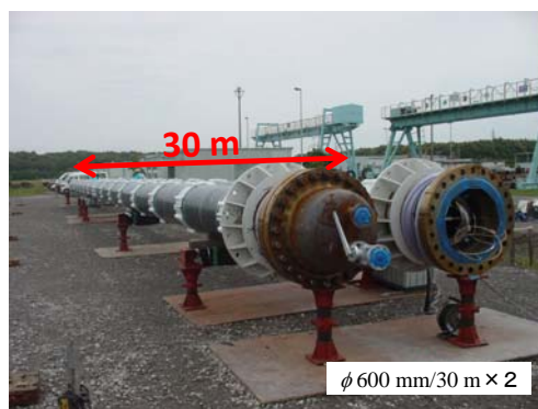
Photo.2 Pipe holders before burial
